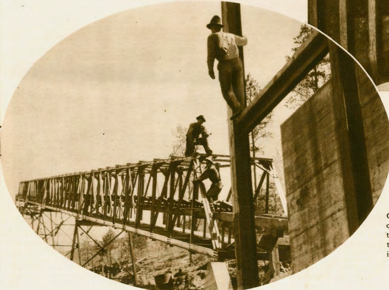
THE SITE of the General Joe Wheeler Dam, also under construction at the present time by TVA, is 15 miles up-stream from Wilson Dam. Wheeler Dam will be 6,400 feet long, 70 feet high. It will provide a storage lake 80 miles long and a potential generating capacity of 375,000 horsepower.
