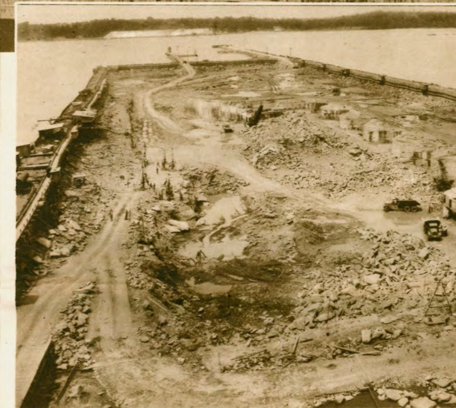
THE SITE of the General Joe Wheeler Dam, also under construction at the present time by TVA, is 15 miles up-stream from Wilson Dam. Wheeler Dam will be 6,400 feet long, 70 feet high. It will provide a storage lake 80 miles long and a potential generating capacity of 375,000 horsepower.
