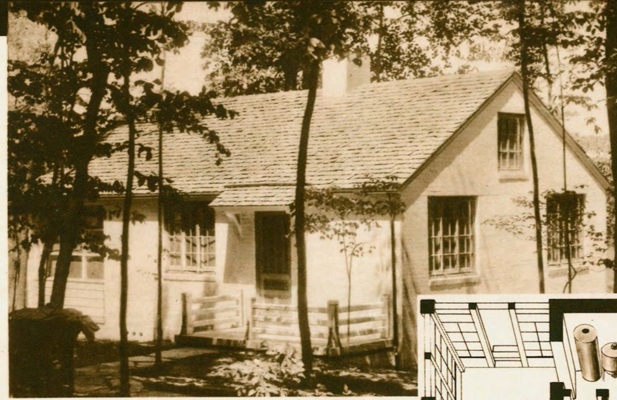
View of an electrified house at Norris, Tennessee. Such a home will rent for about $25 a month. Norris will have 200 to 300 such houses. Some will be larger and rent for a little more. Many will be heated by electricity. All will utilize cheap electricity from the Tennessee River for lights, cooking, refrigeration, and many other household uses.
