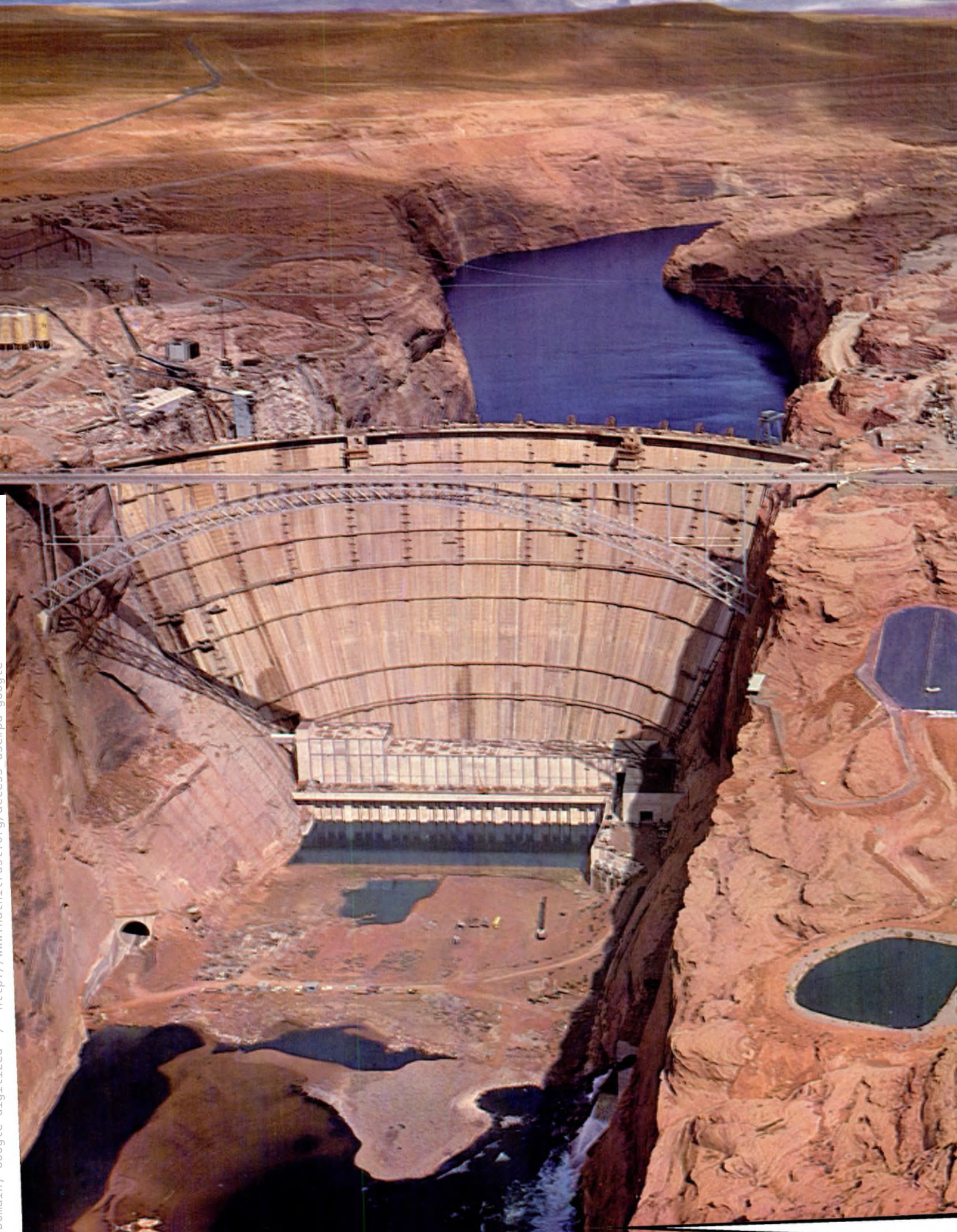
GLEN CANYON DAM— Complete and Storing Blue Water.
